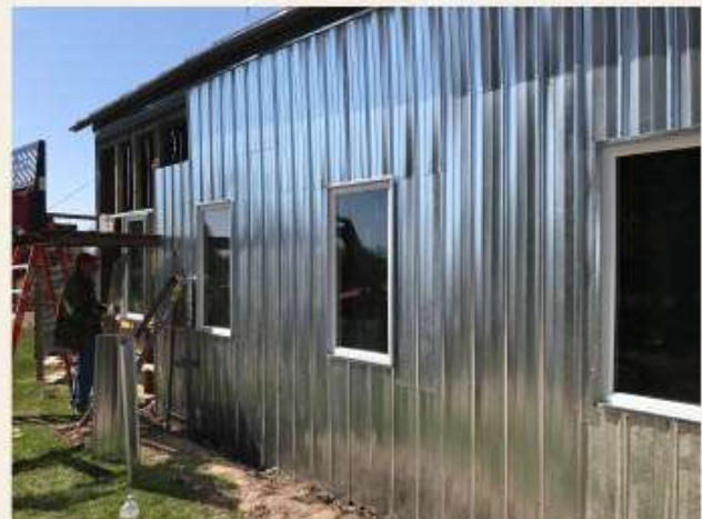
Nate working on the machine shed exterior
