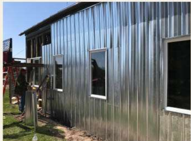
Nate working on the machine shed exterior
