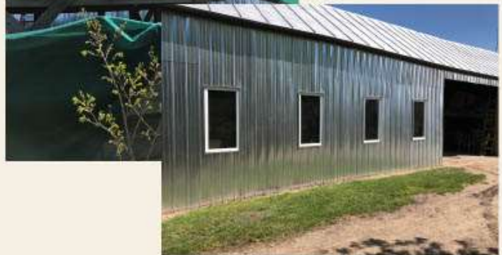
Siding the machine shed with metal
