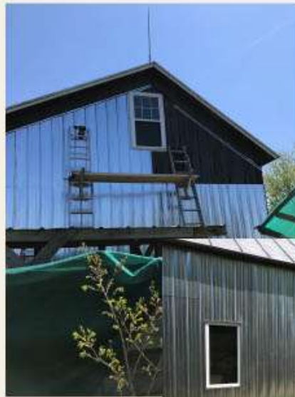
Siding the machine shed with metal
